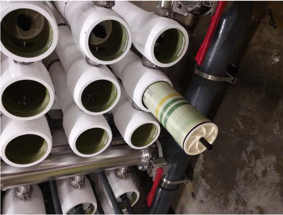
RO membrane element being installed in the pressure vessel located on the skid unit.
