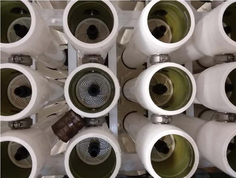
Open end cap of the pressure vessel with an installed RO element. Each skid unit is designed to treat 2.2 million gallons of water per day (MGD).
