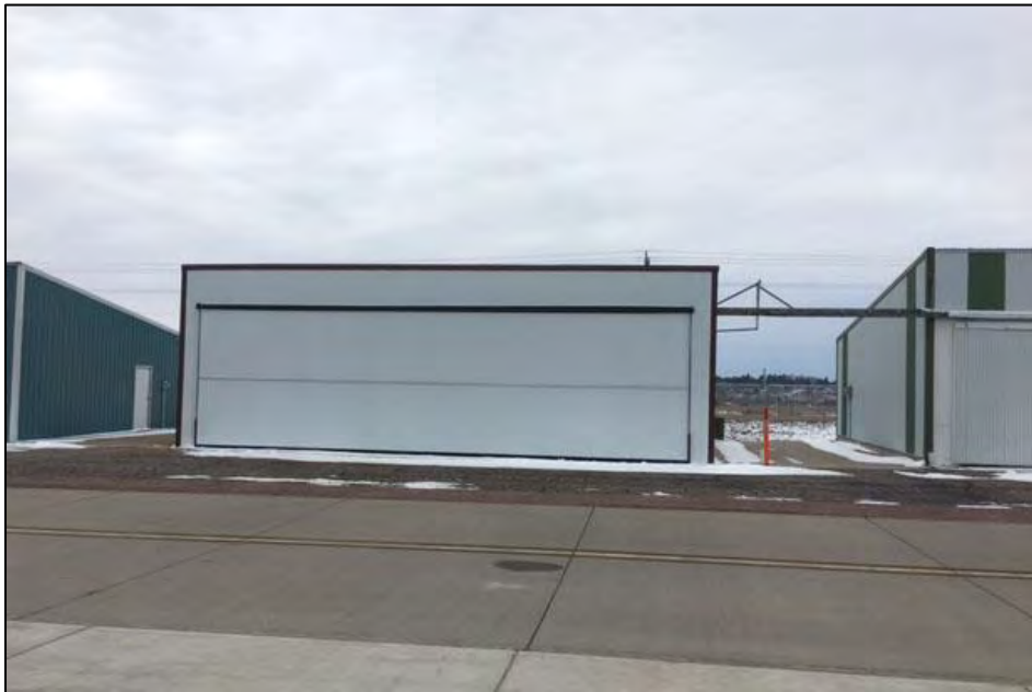
Structure 59911 Structure C15 facing southwest. B. Moloney 3/15/2017.
