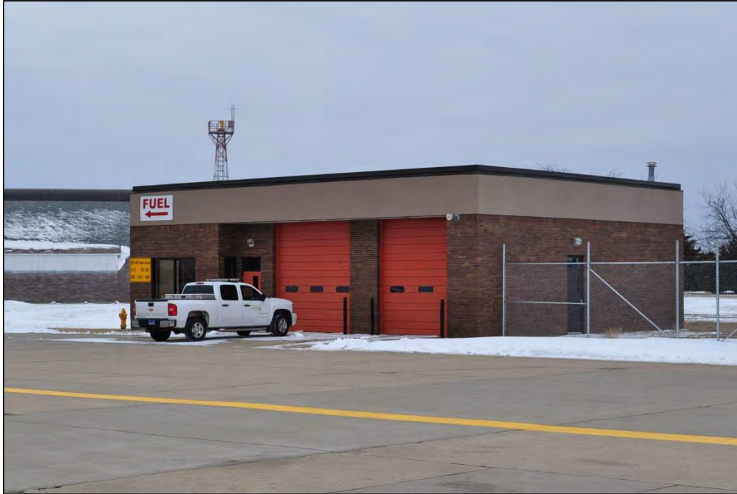
Figure 14. Chan Gurney Airport Fire Station building facing southwest. B. Moloney 3/15/2017.
