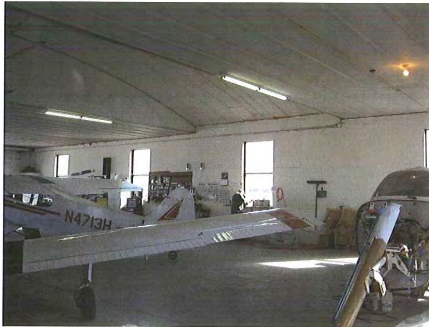
13. Looking at east wall of hangar.
