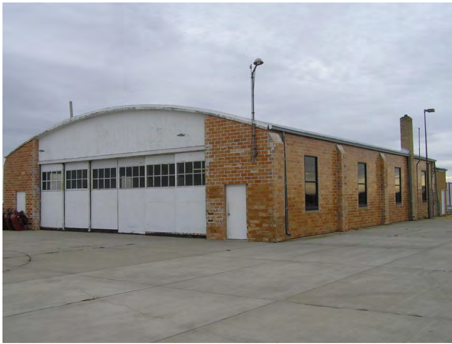
PHOTOGRAPH 1. Building A - 1943 Tile Hangar Building, looking south and east.
