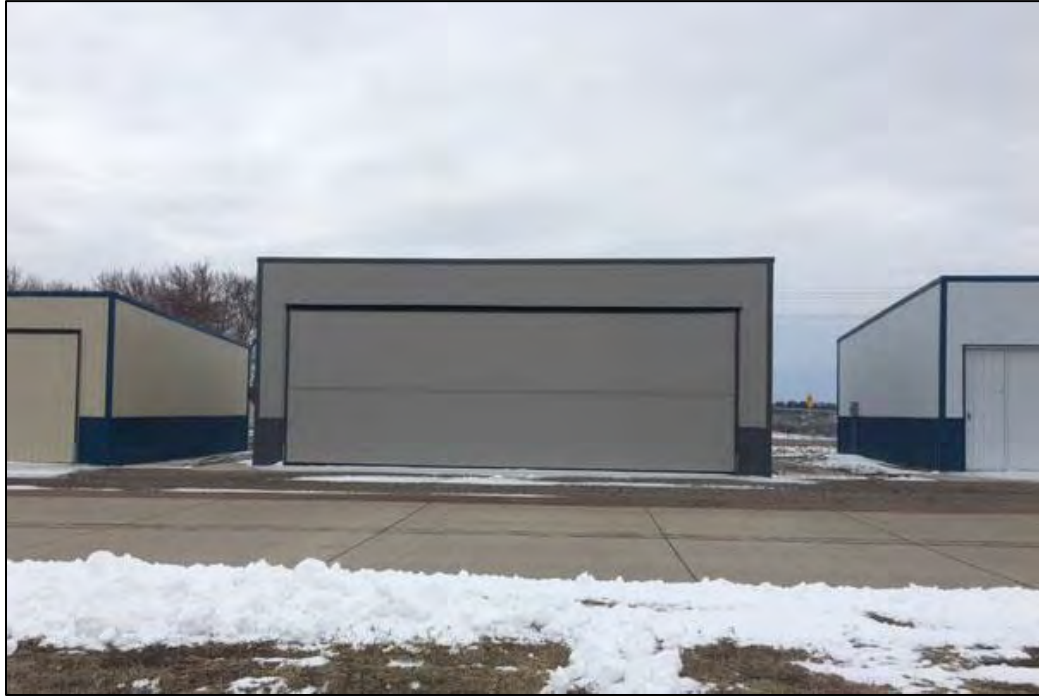
Figure 12. Typical shed roof airplane hangar structure found at Chan Gurney Airport facing west. 27 of the 34 structures surveyed were of this type. B. Moloney 3/15/2017.
