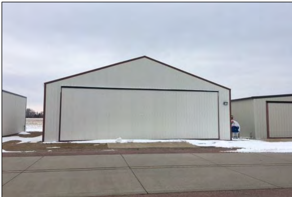
Structure 59901 Structure C5 facing northeast. B. Moloney 3/15/2017.
