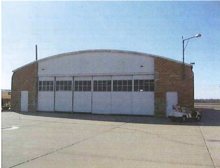
1. Front of hangar faces north.
