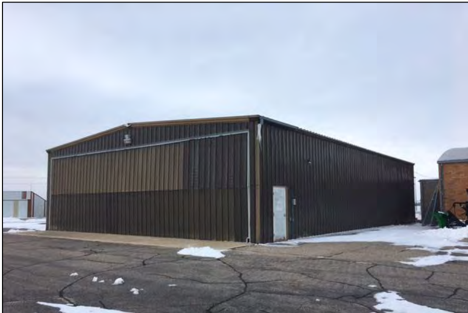
Structure 59895 Structure B facing southeast. B. Moloney 3/15/2017.
