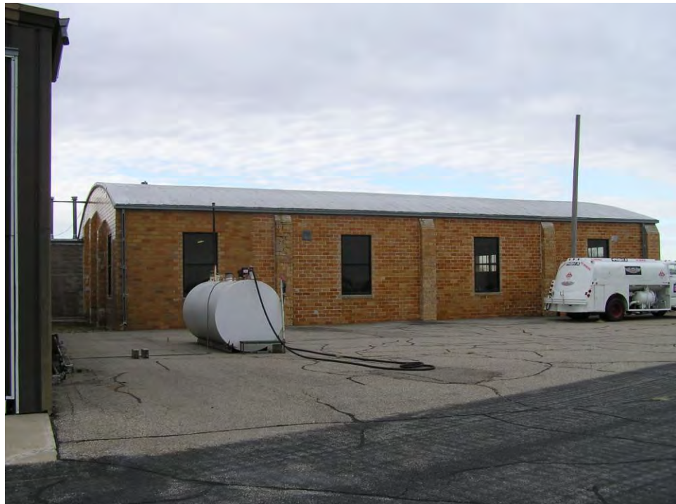
PHOTOGRAPH 3. Building A - 1943 Tile Hangar Building, looking west. Note the modification to the window openings and different appearance of the clay tile to the building's rear.
