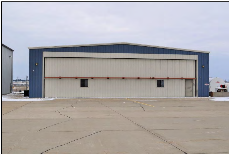
Structure 59891 Structure K facing west. B. Moloney 3/15/2017.
