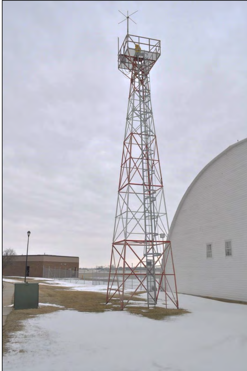
Figure 11. Structure O Radio Tower facing northeast. B. Moloney 3/15/2017.
