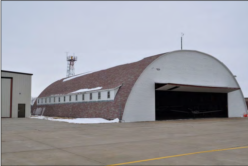
Figure 7. Arched roof barrel hangar looking northwest. B. Moloney 3/15/2017.
