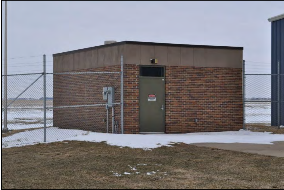
Structure 59892 Structure L facing northeast. B. Moloney 3/15/2017.
