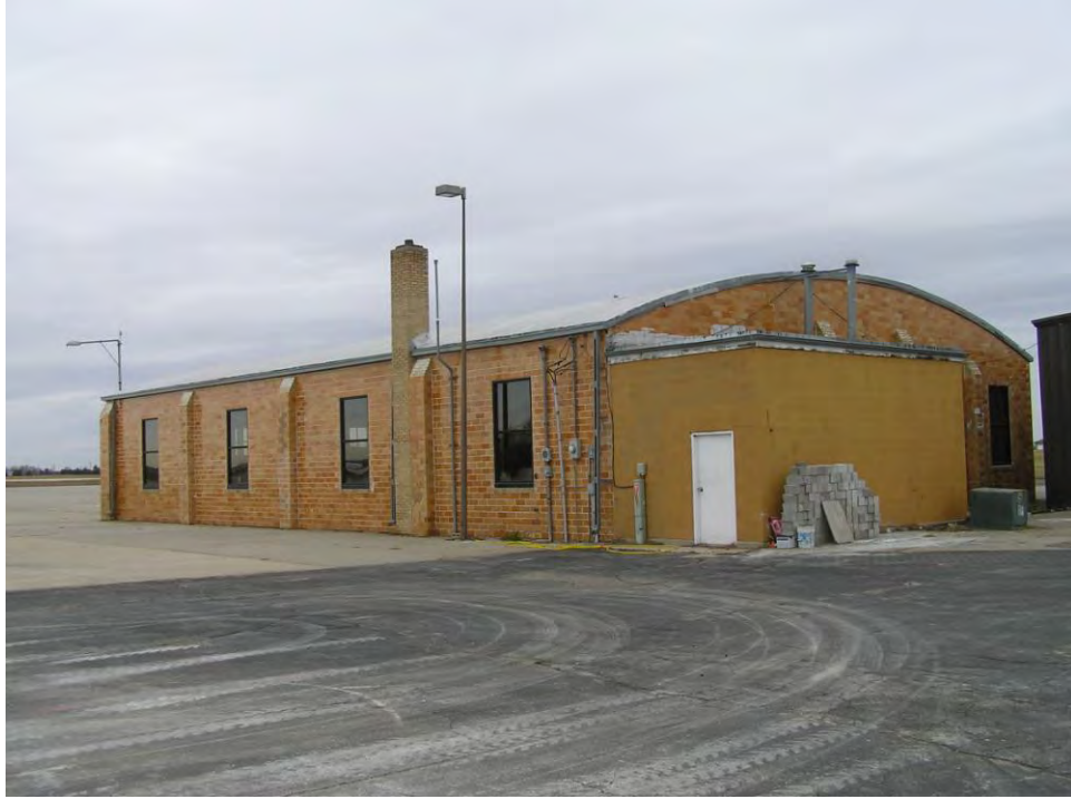
PHOTOGRAPH 2. Building A - 1943 Tile Hangar Building, looking north and east.
