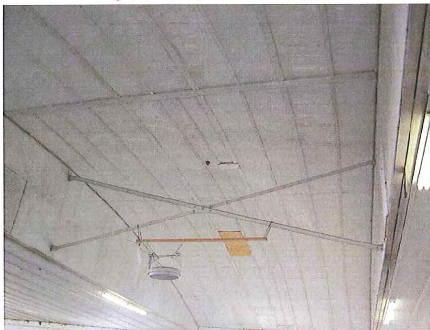
24. Steel cross bracing at midspan between bowstring trusses.
