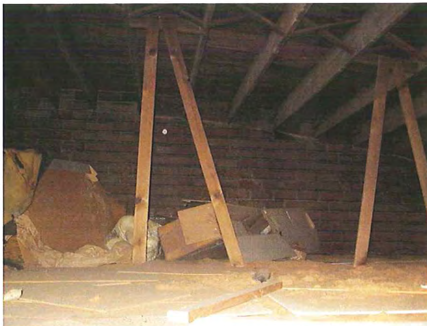
23. Attic looking south. 2x12 joists bear on south wall of hangar.
