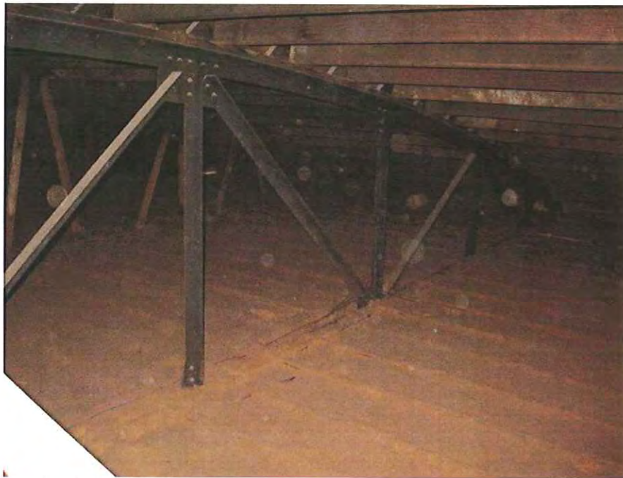
22. East side of bowstring truss.
