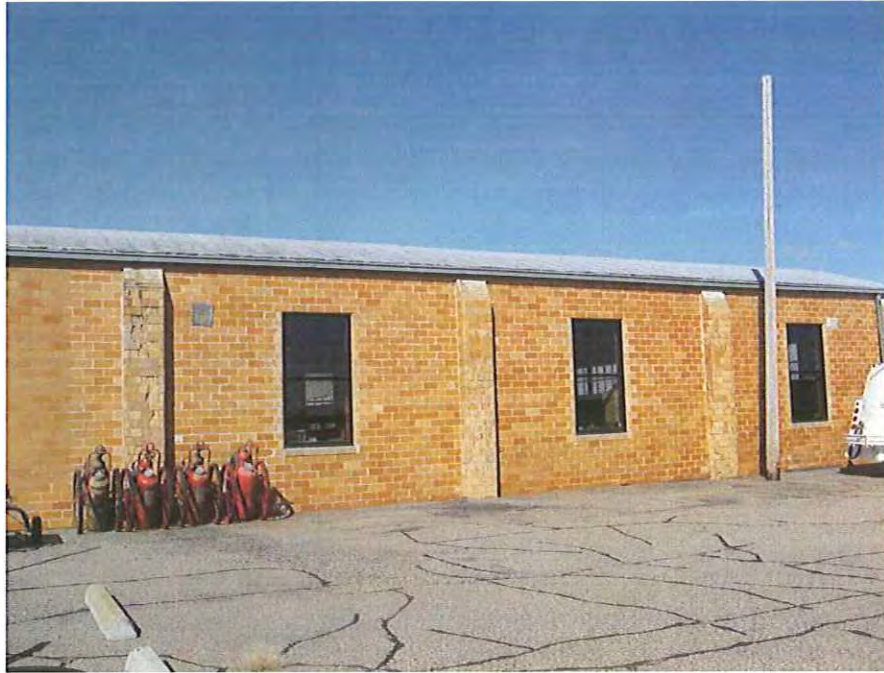
3. East side of the hangar.
