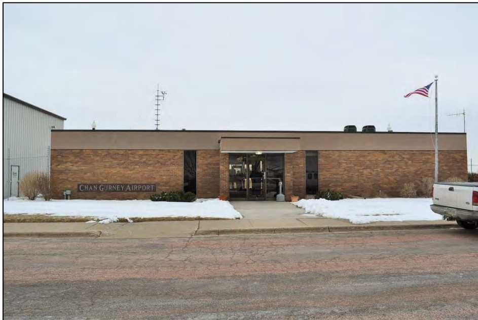
Structure 59889 Structure I Terminal facing east. B. Moloney 3/15/2017.
