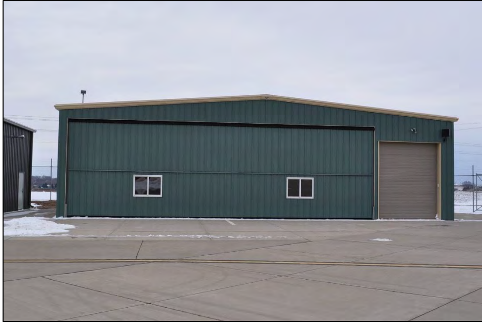
Structure 59886 Structure E facing west. B. Moloney 3/15/2017.
