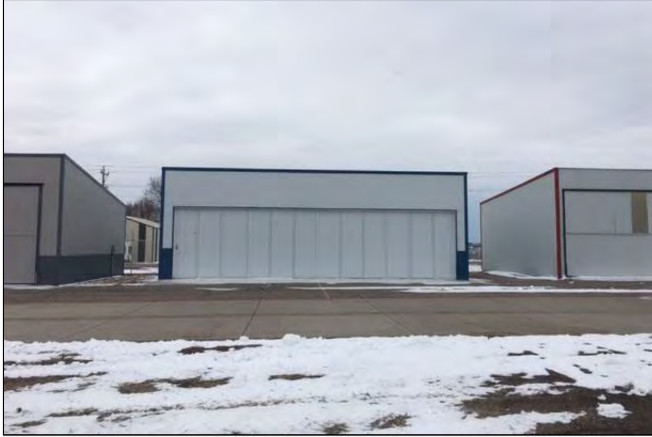
Structure 59906 Structure C10 facing southwest. B. Moloney 3/15/2017.
