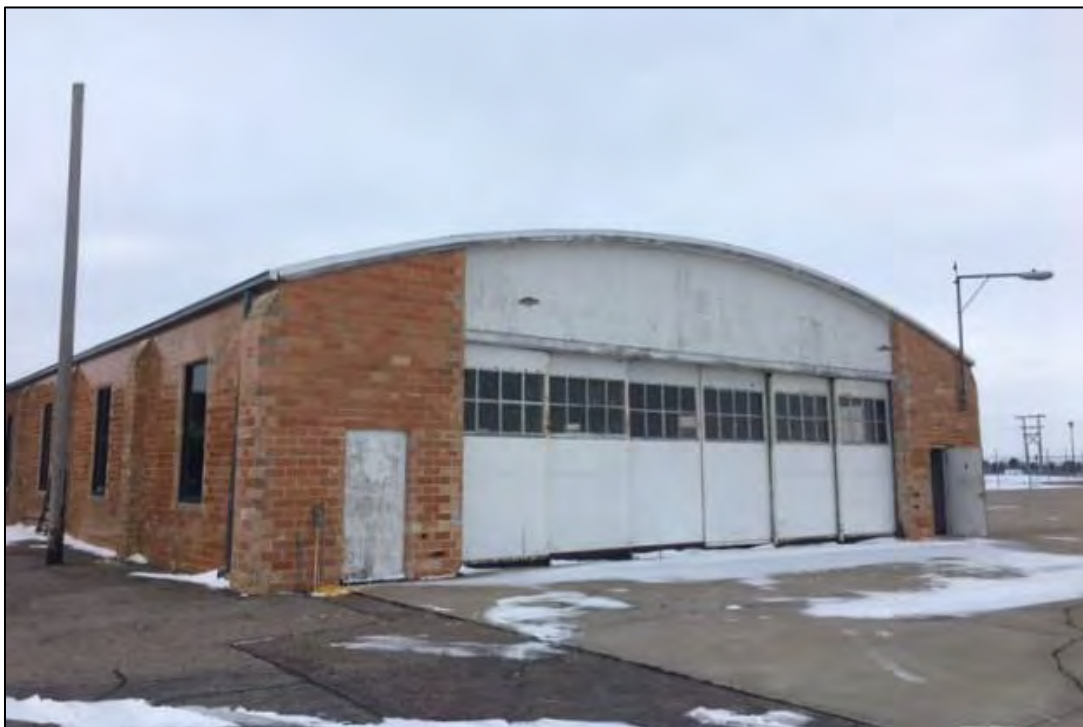
Figure 6. Condition of tile hangar as observed during 2017 survey. B. Moloney 3/15/2017.
