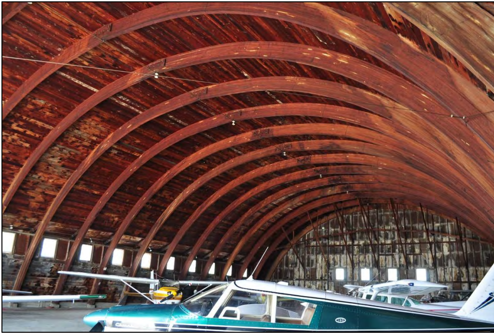
Figure 10. Interior view of the barrel hangar showing structural arches and west wall with steel support beams. B. Moloney 3/15/2017.
