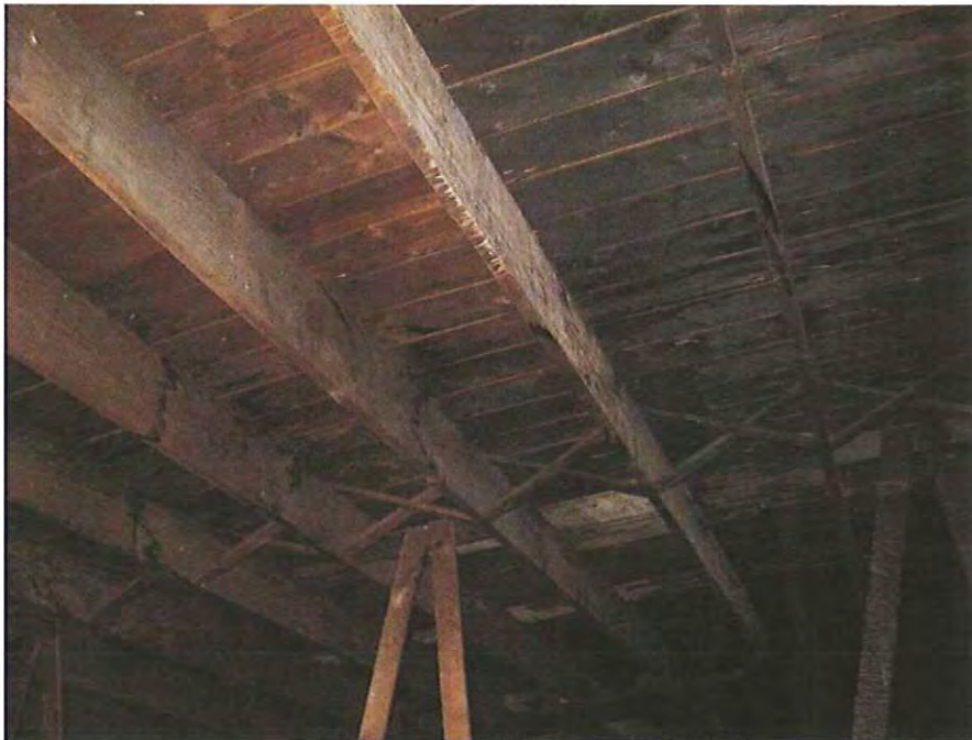
20. 2x12 wood joists and bracing supporting roof decking.
