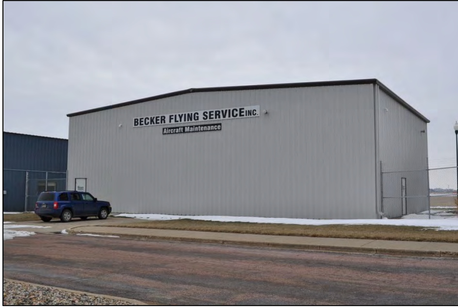
Structure 59890 Structure J facing northeast. B. Moloney 3/15/2017.
