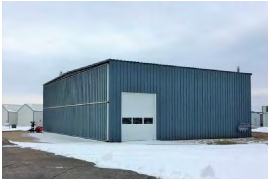
Structure 59897 Structure C1 facing southwest. B. Moloney 3/15/2017.
