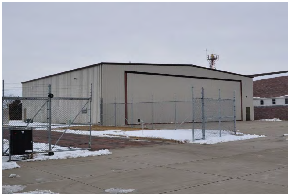
Structure 59885 Structure F facing northwest. B. Moloney 3/15/2017.
