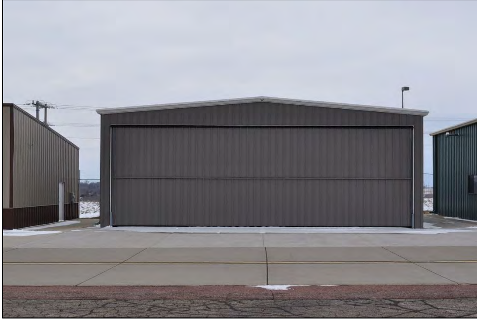
Structure 59916 Structure C20 facing southwest. B. Moloney 3/15/2017
