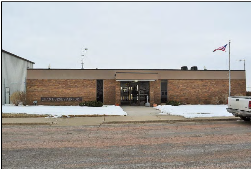
Figure 13. Chan Gurney Airport terminal building facing east. B. Moloney 3/15/2017.
