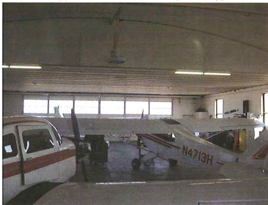
12. Looking at north wall of hangar.
