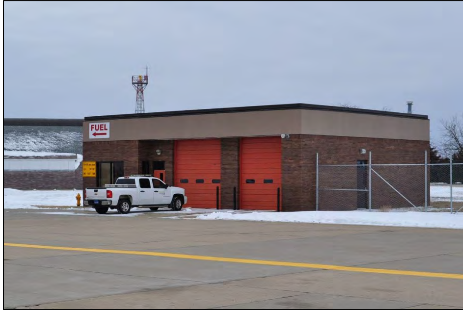
Structure 59888 Structure Fire Station facing southwest. B. Moloney 3/15/2017.
