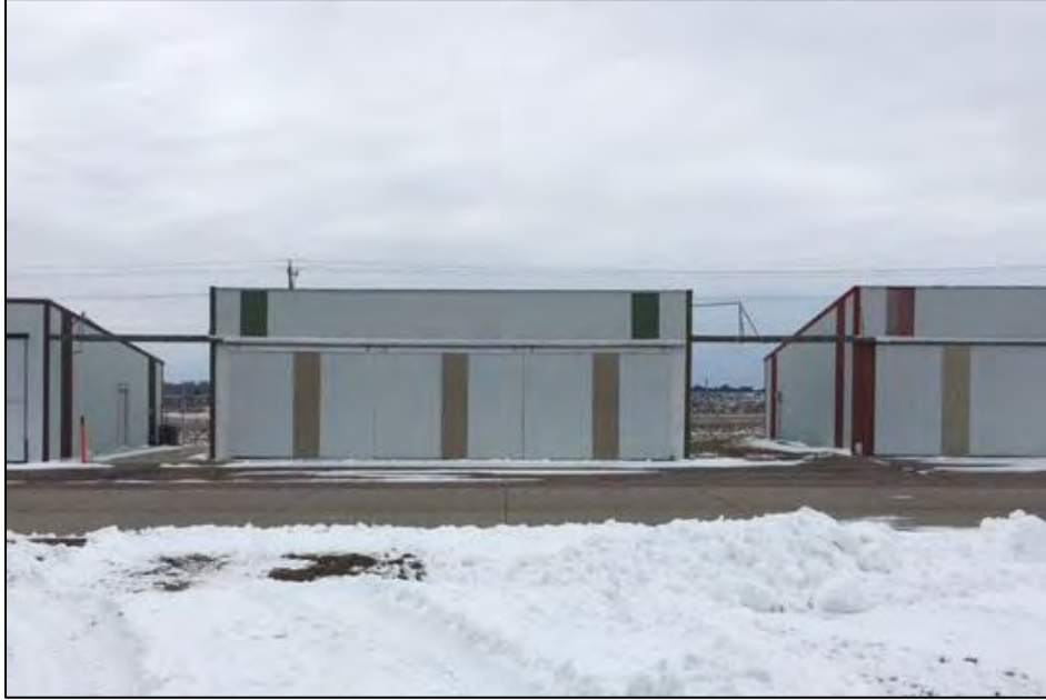
Structure 59912 Structure C16 facing southwest. B. Moloney 3/15/2017.
