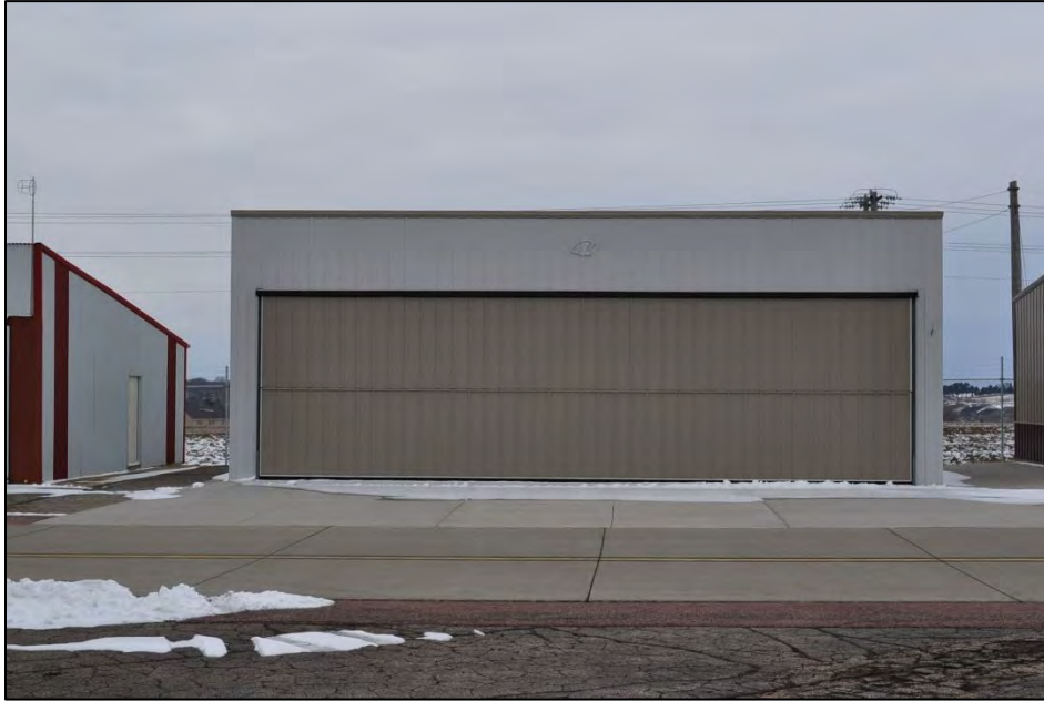
Structure 59914 Structure C18 facing southwest. B. Moloney 3/15/2017.
