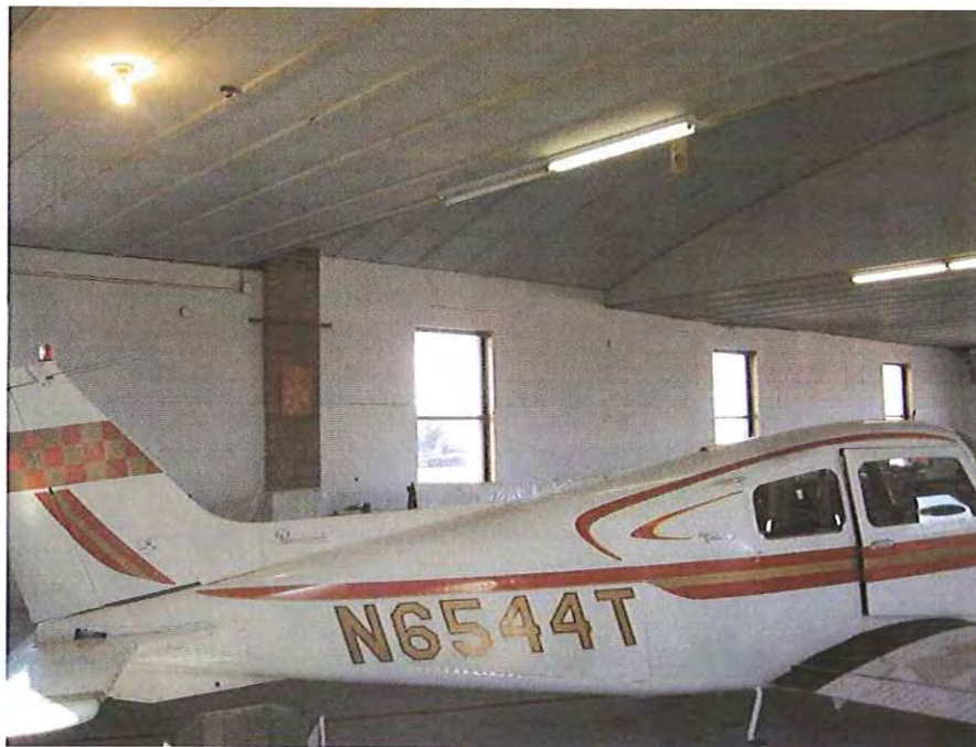
14. Looking at west wall of hangar.
