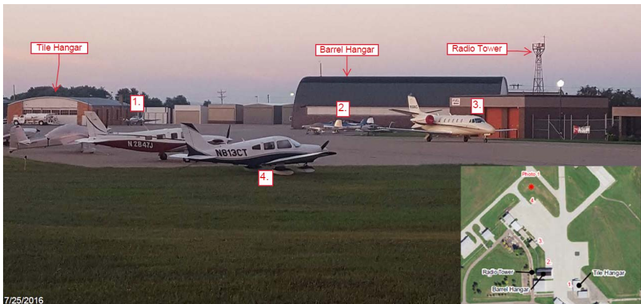
1. Aircraft parked in an unsuitable parking area. 2. ADG I aircraft parked in the large aircraft parking area. 3. ADG II aircraft parked in loading and unloading area. 4. All parking tiedowns being used by ADG I aircraft.
