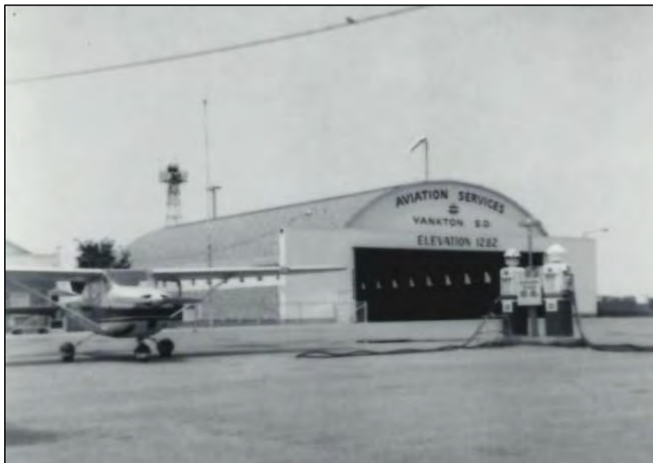
Figure 2. 1940s historic photo of the Chan Gurney barrel hangar showing the original sliding doors on the building's east elevation. Notice the radio tower in the background as well. Photo courtesy of Mike Roinstad, Chan Gurney Airport Supervisor.
