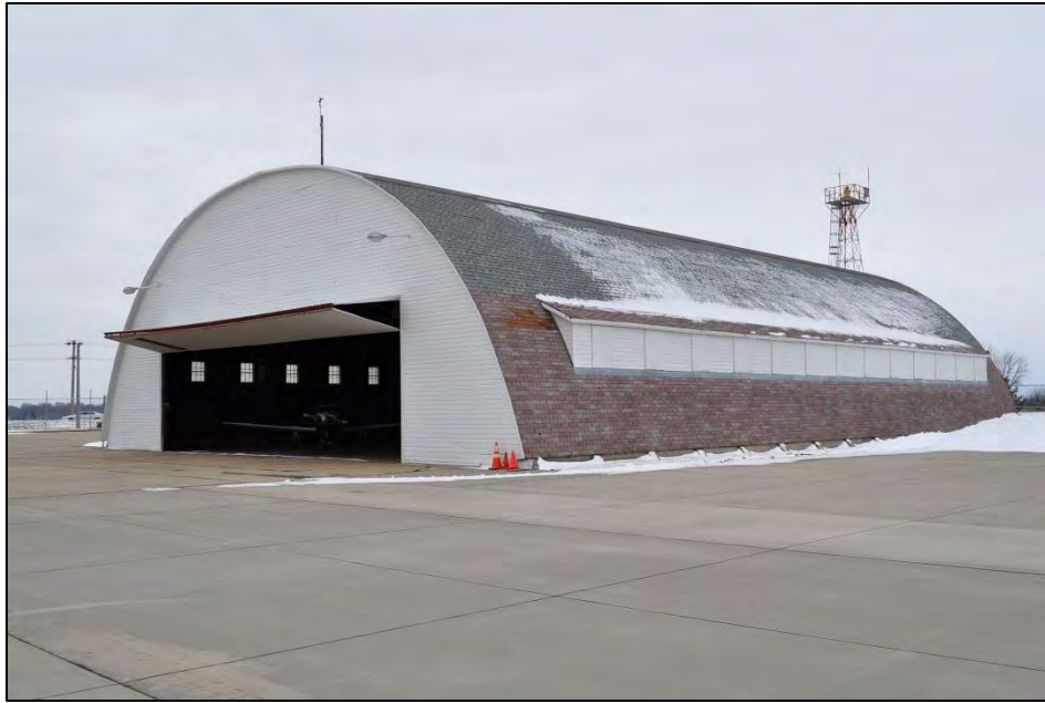
Structure 59884 Structure G Barrel Hangar facing southwest. B. Moloney 3/15/2017.
