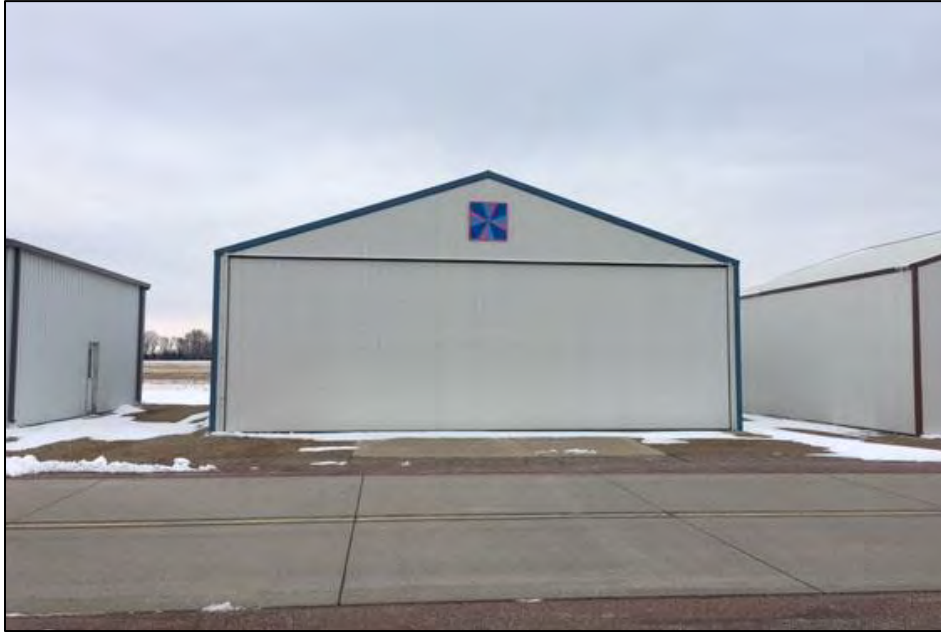
Structure 59900 Structure C4 facing northeast. B. Moloney 3/15/2017.
