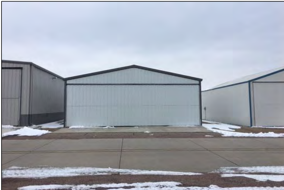
Structure 59899 Structure C3 facing northeast. B. Moloney 3/15/2017.
