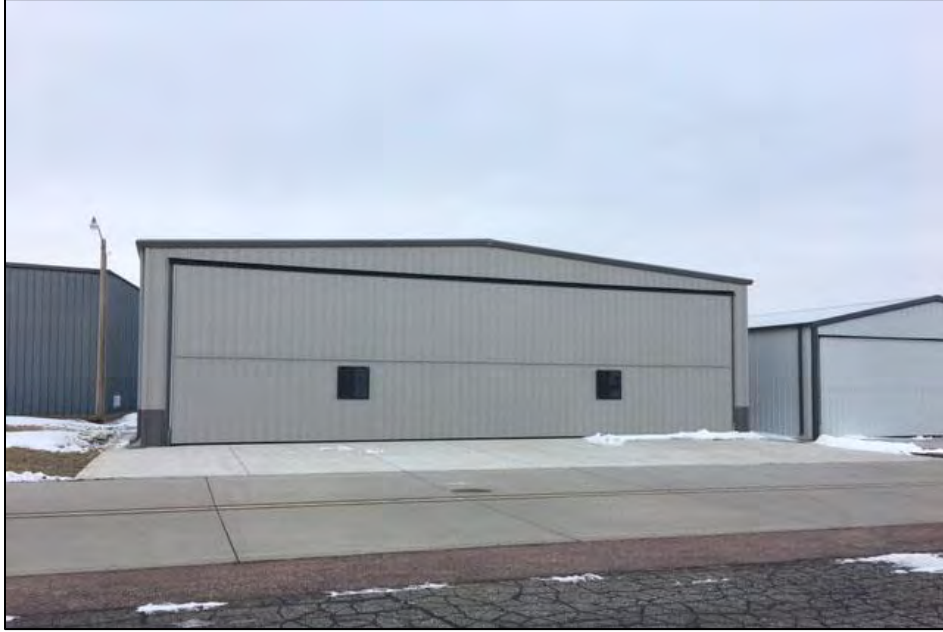
Structure 59898 Structure C2 facing northeast. B. Moloney 3/15/2017.
