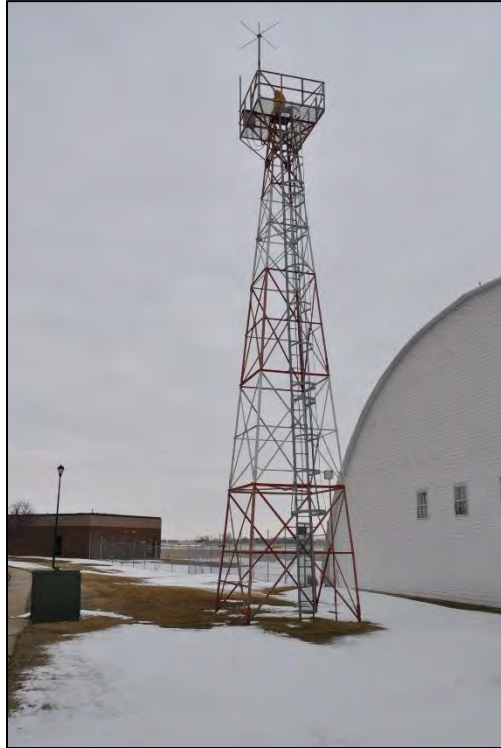
Structure 59896 Structure O Radio Tower facing northeast. B. Moloney 3/15/2017.
