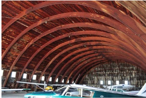
Photo 2, Based Aircraft Inside Barrel Hangar
