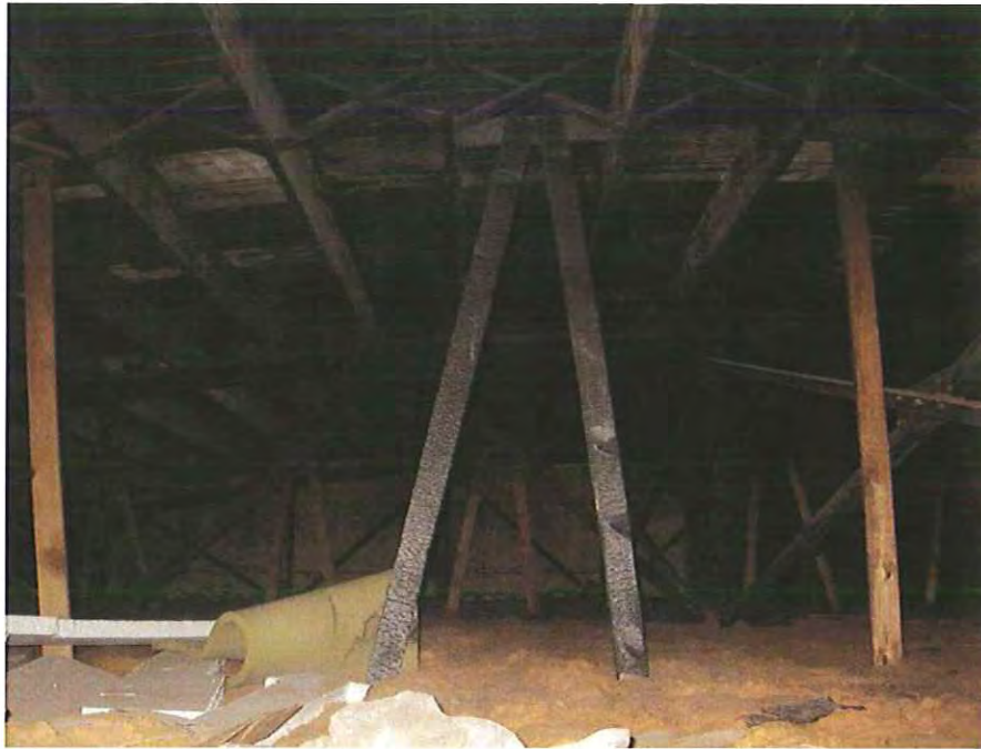
19. Attic looking north.
