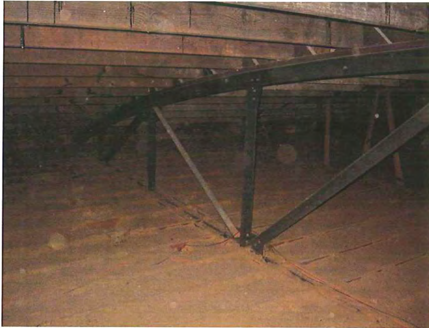
21. West side of bowstring truss.
