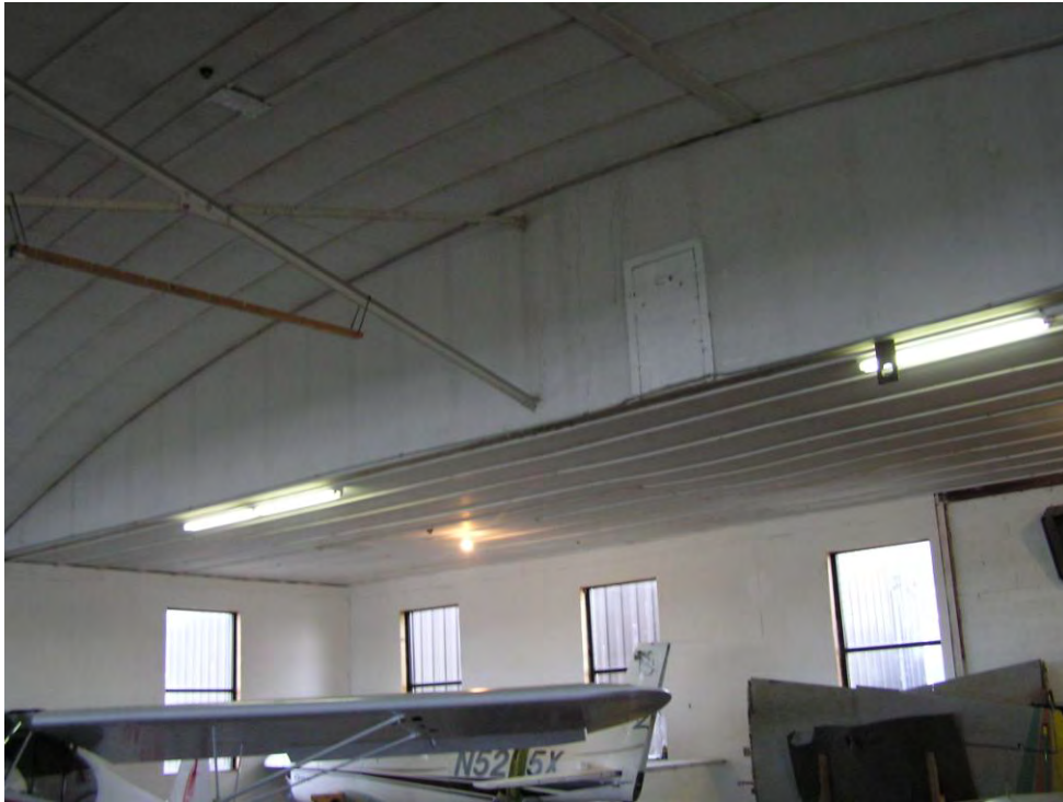
PHOTOGRAPH 6. View of Building A interior ceiling space and 1973 ceiling sheathing.
