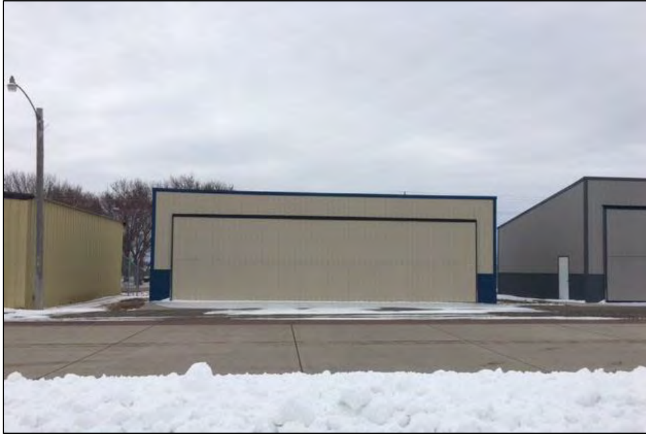
Structure 59904 Structure C8 facing southwest. B. Moloney 3/15/2017.
