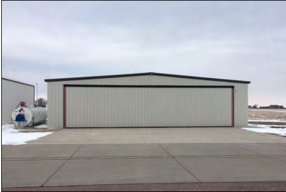
Structure 59902 Structure C6 facing northeast. B. Moloney 3/15/2017.
