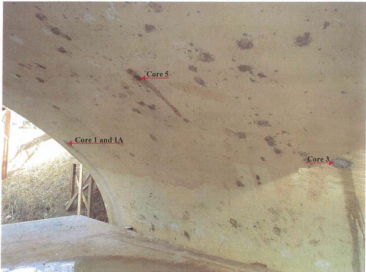
Image 21: Location of arch cores 1, 1A, 3 and 5 looking northwest
