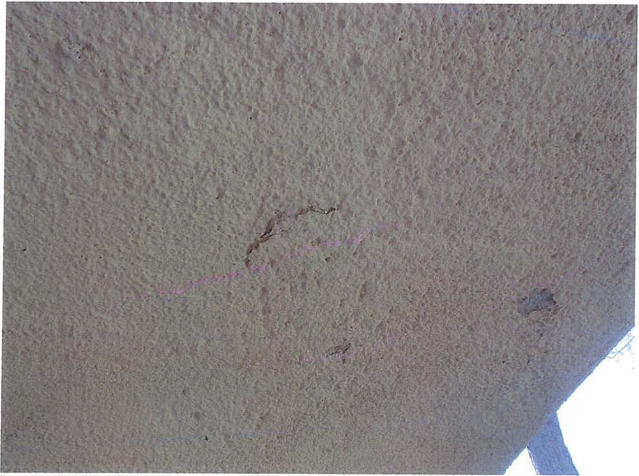
Image 7: Scaling of shotcrete south side of the arch apex, west side of arch
