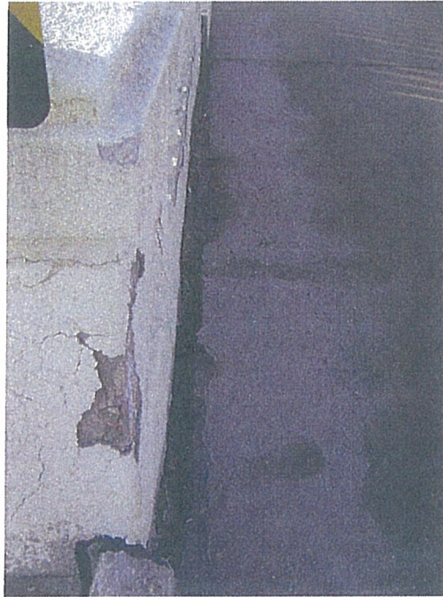
Photo 6: Gap between PCCP Deck and Vertical Side Wall at Northeast Corner of Bridge
