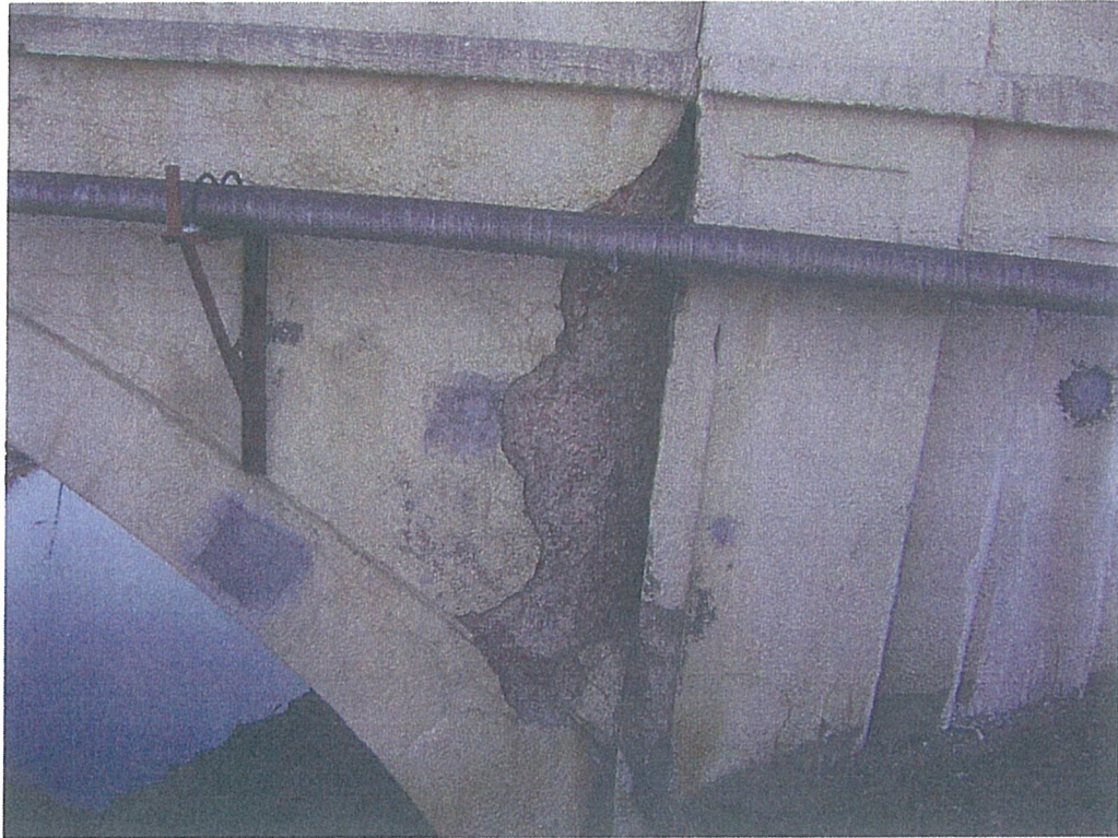
Photo 8: Deterioration of Concrete at Construction Joint at Southwest Corner of Arch
