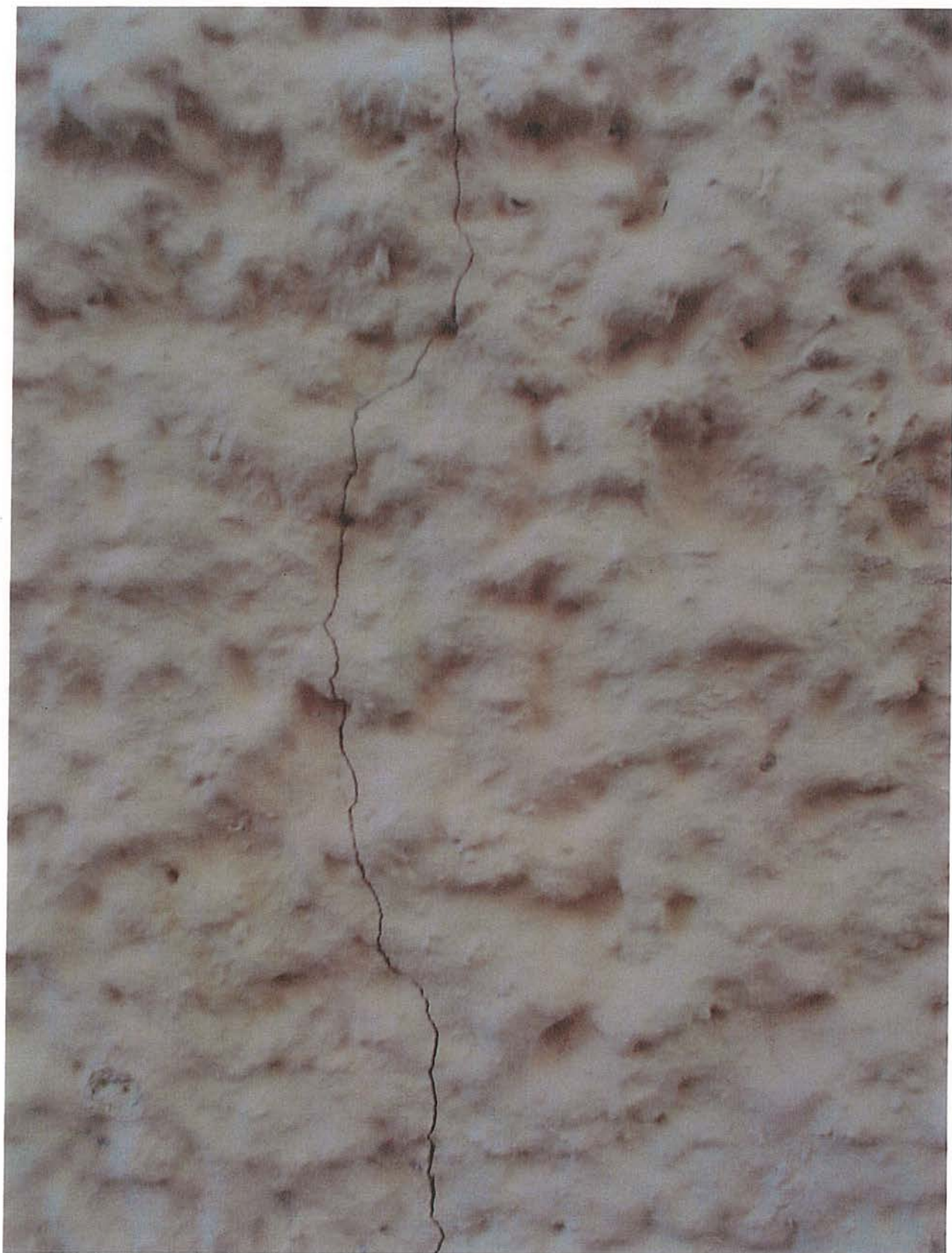
Image 6: Crack near the location of arch core 2
