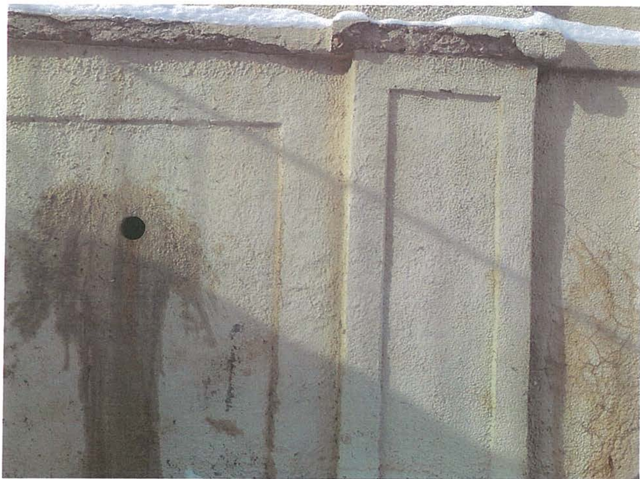
Image 13: Location of the core sample from the southeast wall
