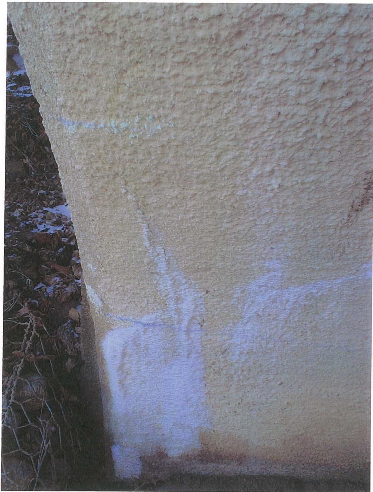
Image 4: Crack and efflorescence staining at southeast corner of the arch
