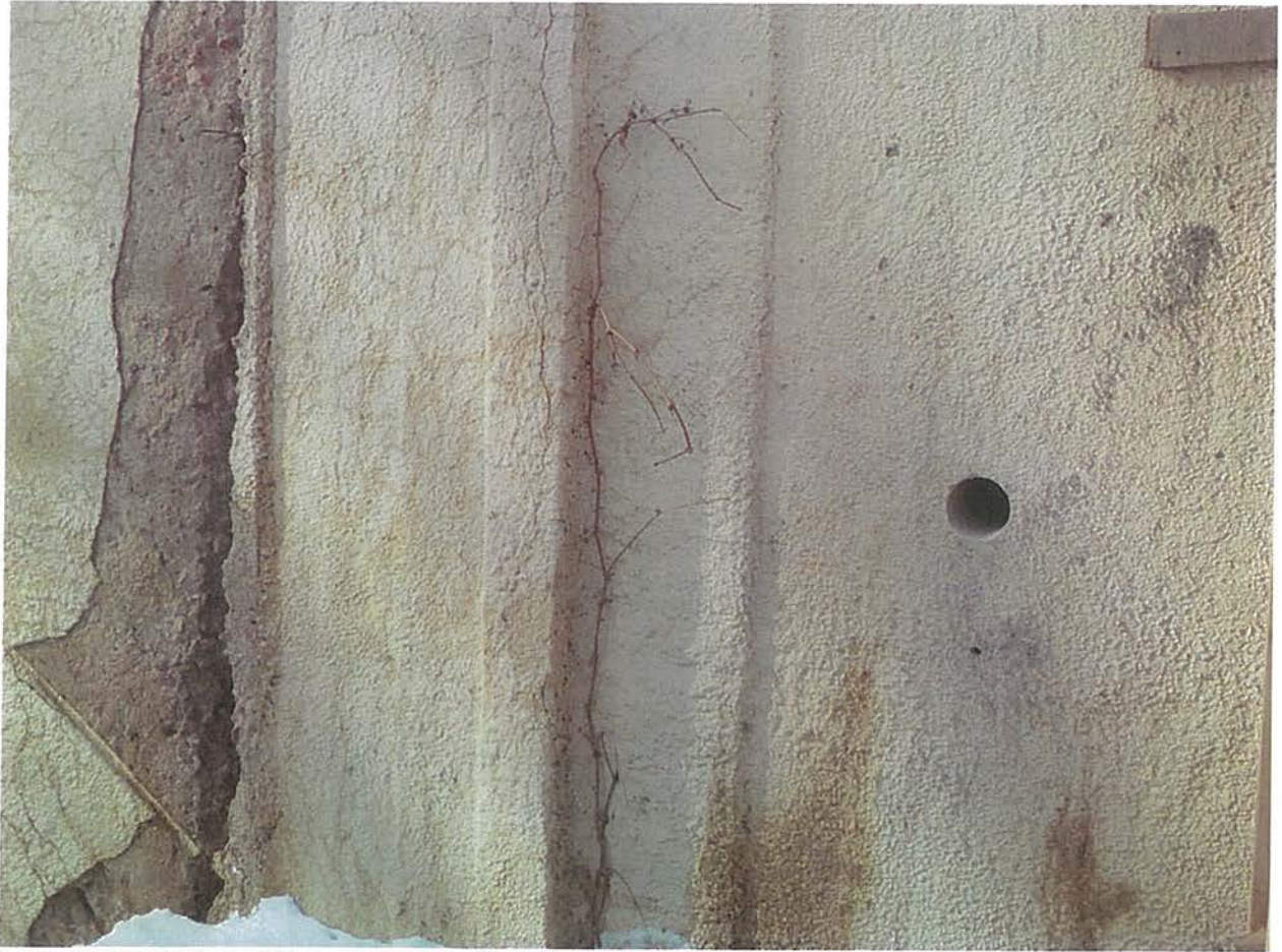
Image 11: Location of the core sample from the northeast wall
