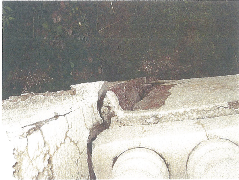
Photo 9: Out of Plumb Elements and Deterioration of Concrete at Construction Joint at Northeast Corner of Arch (looking down)
